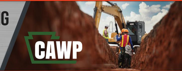
Excavations can be extremely dangerous. That's why OSHA requires a competent person to oversee all excavation and trenching operations. The competent person must have specific training in – and be knowledgeable about – soil analysis, the use of protective systems, and the requirements of OSHA's excavation standard.
