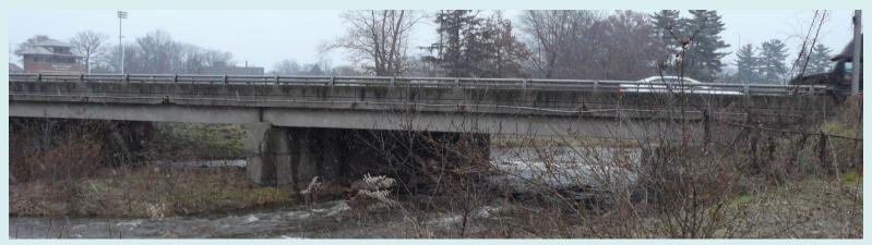
Superstructure Replacement: existing spread box beam with minor approach roadway work under half-width construction. (134')
