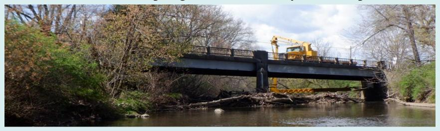
**Replacement:** Single span, prestressed, concrete bulb tee-beam on reinforced concrete cantilever abutments bridge, pier removal, guide rail and paving; (135')
