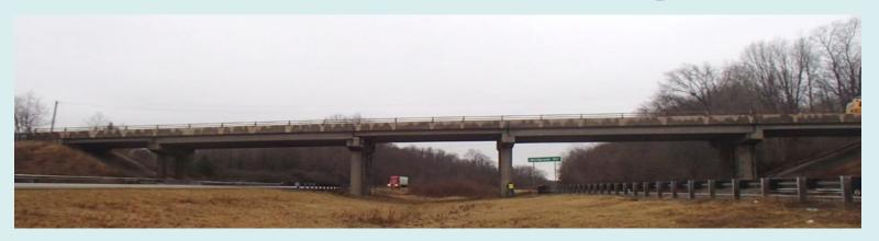
**Preservation:** concrete deck, tying the deck together at the piers to make a continuous structure, repairs pre-stressed concrete box beams, and repair deteriorated concrete, milling, and paving (232'-5 spans)
