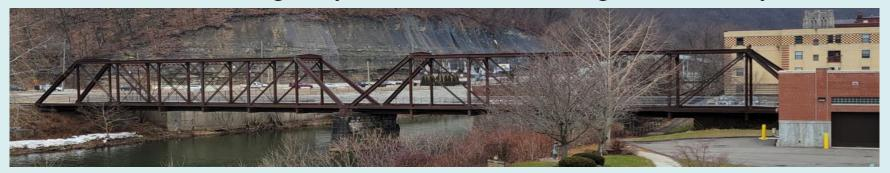
**Bridge Rehabilitation:** hydro-demo, latex overlay, concrete barrier, jacking of superstructure for bearing and pedestal repair/replacement, clean and paint beam ends, replace deck joints, substructure repairs, drainage, new LED lighting. (1,012')
