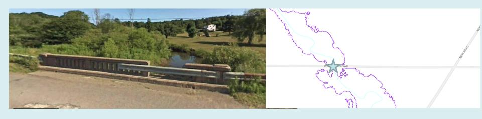
**Restoration:** (35') milling, concrete deck repairs, streambed paving, GRS behind both abutments and overlay of existing tar & chip
